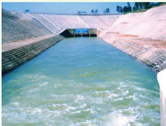
Chennai Water Project
